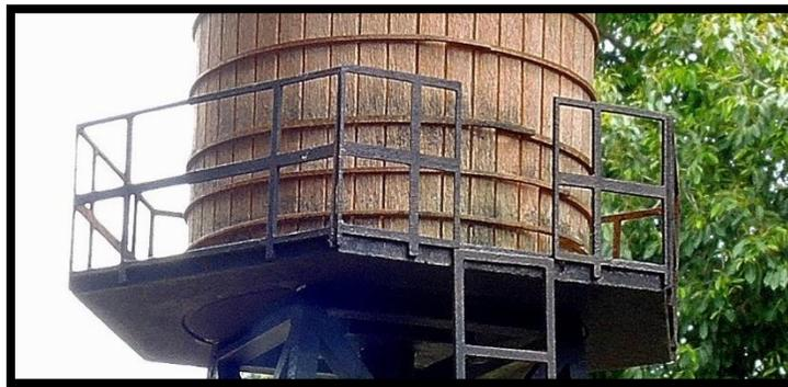
FIGURE #6 –HANDRAILS
